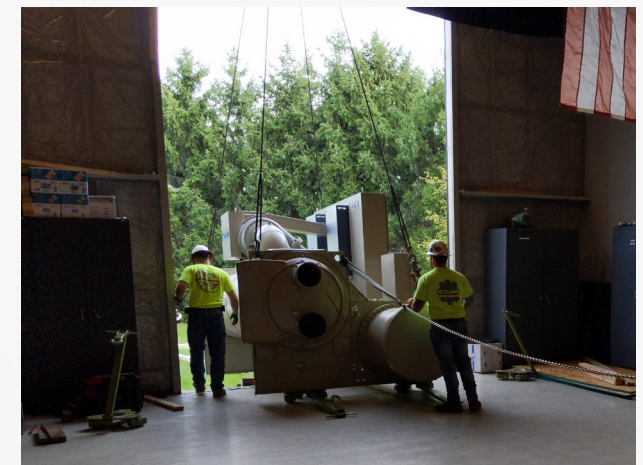
Magnitude chiller unit being lowered on site with additional crane rigging for assistance
